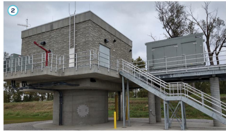
Horizontal collector well similar to what would be constructed near the Missouri River
